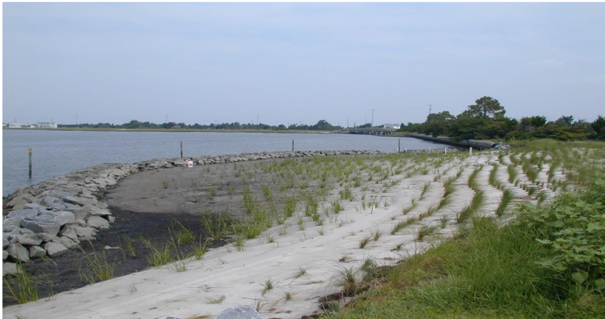
Figure 2. Duke Marine Lab Living Shoreline shortly after construction and planting.
