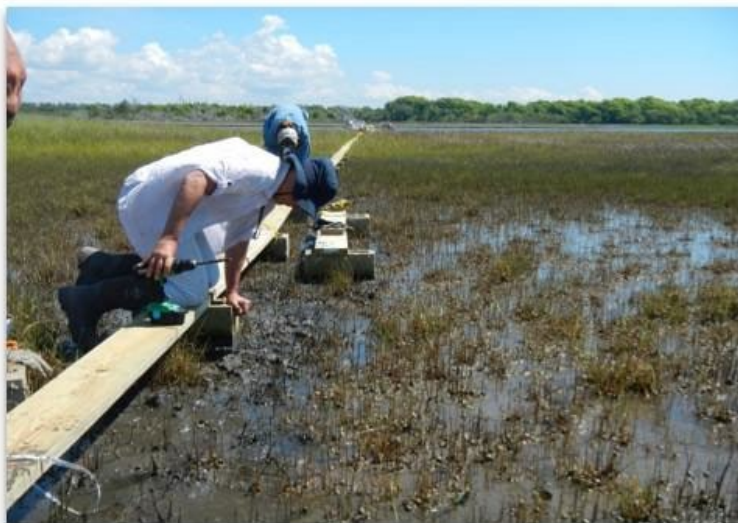
Figure 8. NCCOS staff install temporary boardwalks to minimize impacts to vegetation during sampling.
