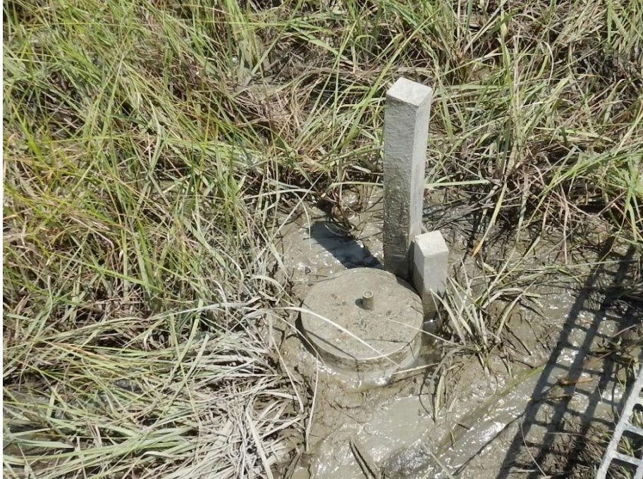
Figure 12. Installation of an elevation benchmark. Diameter of PVC collar is 6", and steel rod can be seen centered in the concrete inside the collar. A Class B or SET benchmark would have an additional stainless-steel fitting around the metal rod to accommodate the SET during readings (see Figure 10).
